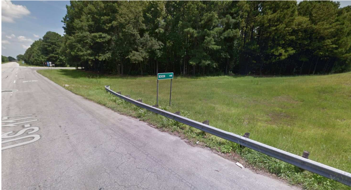
Figure 3.22 I-40 at U.S. 117 Northbound On-Ramp Looking North on U.S. 117
