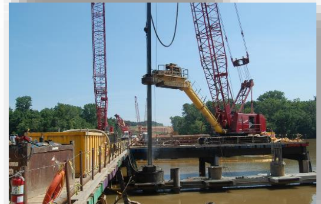
Construction on I-85 bridge over Yadkin river. NCDOT (2011)
