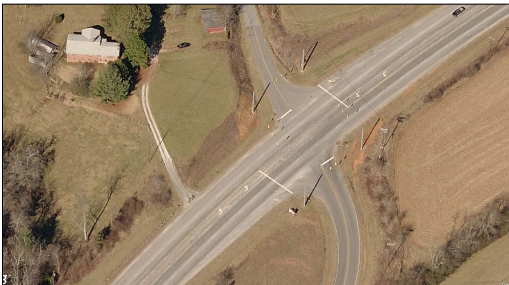
Figure 4.4 NC 280 at Ray Hill Road, Mills River, NC (NC Signal #14-1137)
