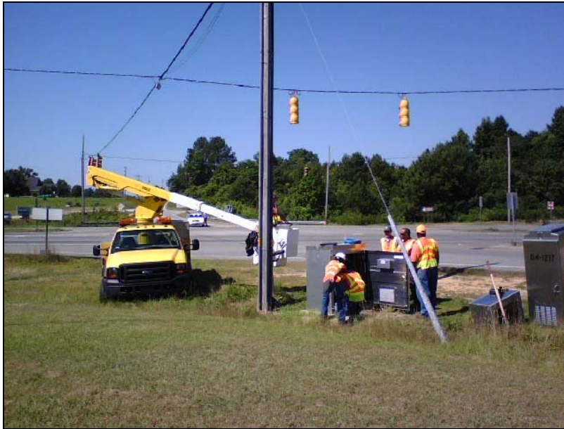
Figure 4.20 Swapping Out the Cabinet and Controller at US 70 and Swift Creek
