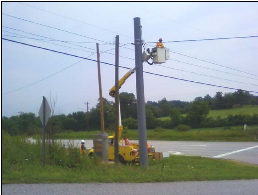
Figure 4.24 Installing the Access Point at NC 280 and Ray Hill Road
