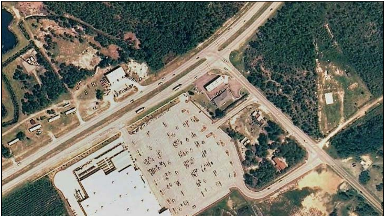
Figure 4.6 US 17 at NC 210, Surf City, NC (NC Signal #03-0618)
