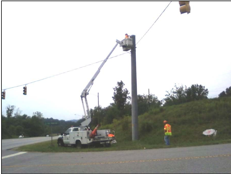
Figure 4.23 Installing the Bounce Repeater at NC 280 and Ray Hill Road
