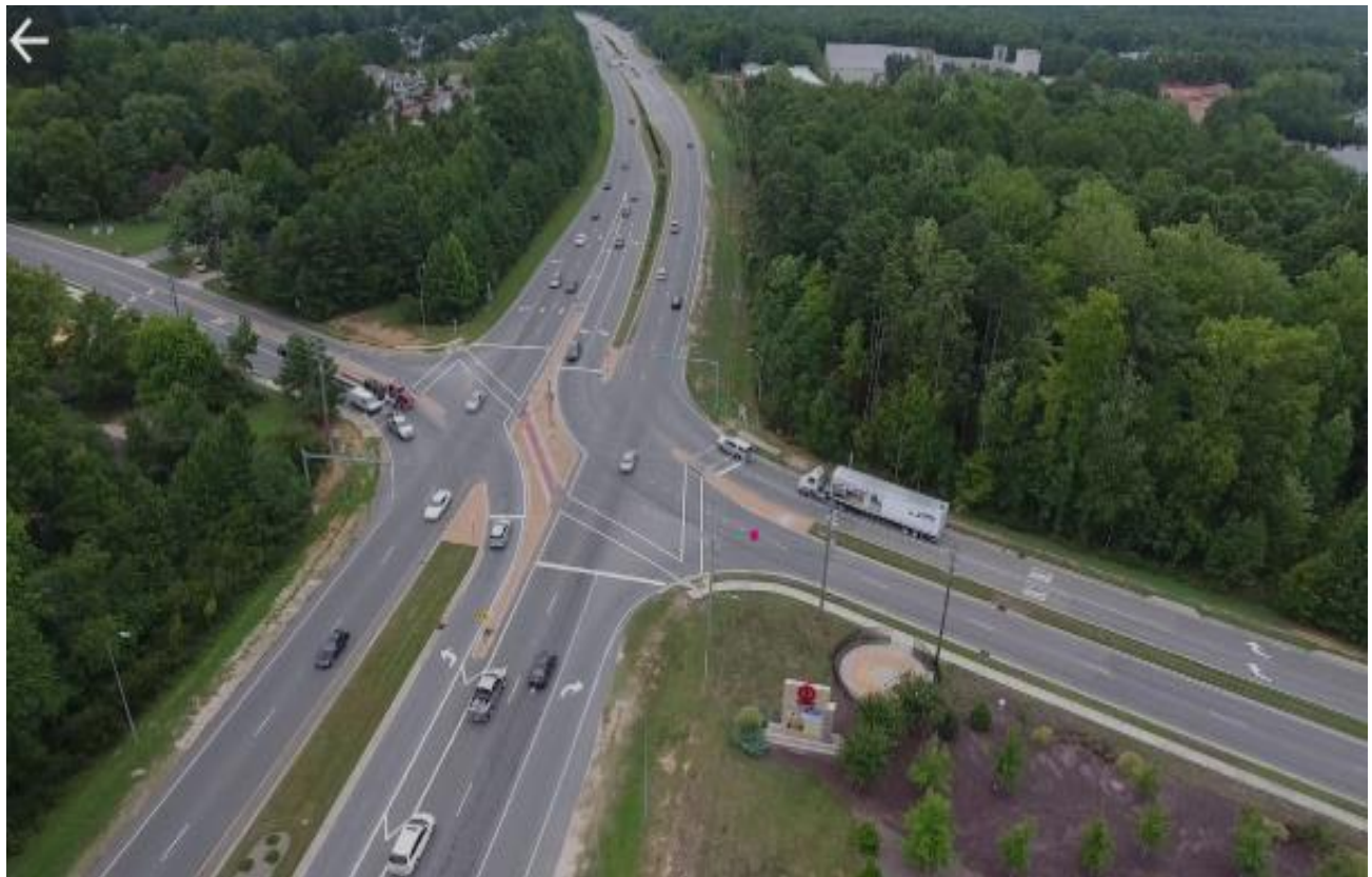
Figure 10-1: Reduced Conflict Intersection / NC-55 & Holly Springs Road / New Hill Road / 35°39'27.86"N / 78°50'54.99"W
