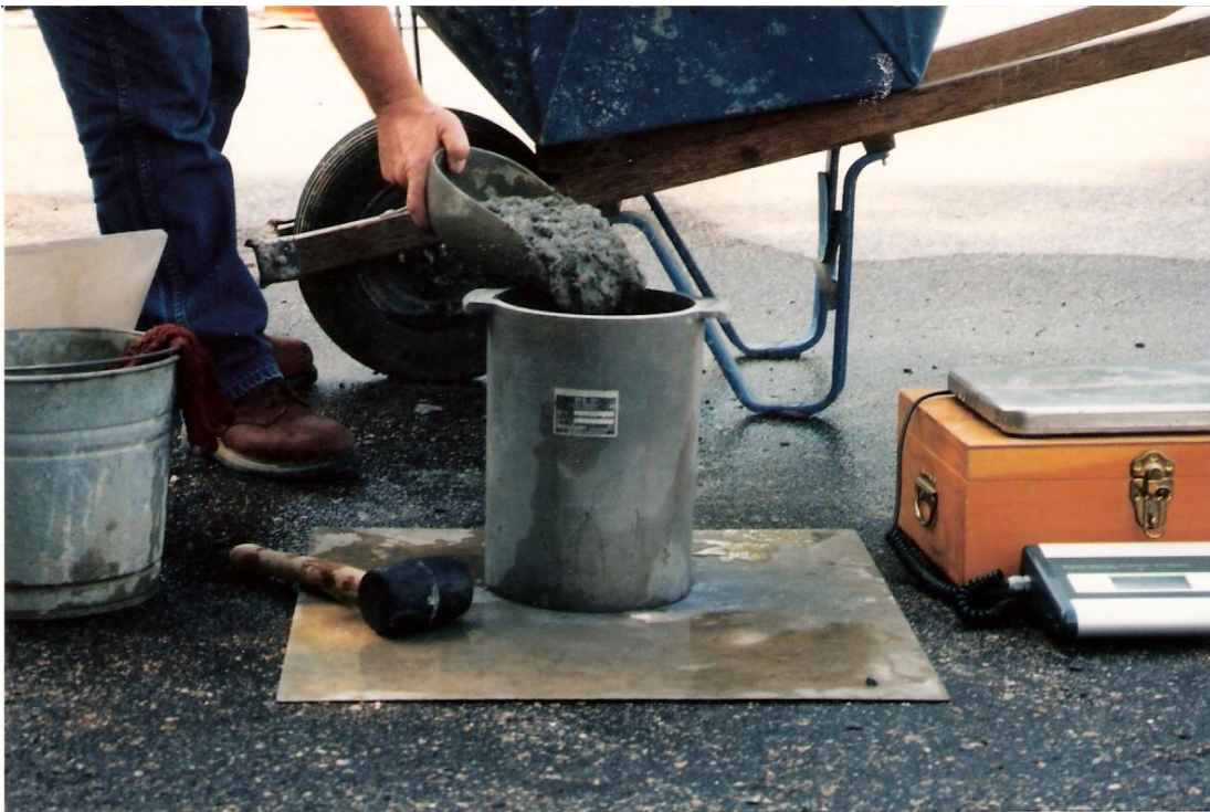
The second layer is to be filled to approximately \frac{2}{3} of the measure volume, distributing concrete evenly.
