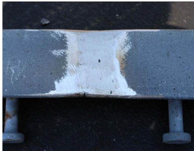
The completed weld is grinded flush
