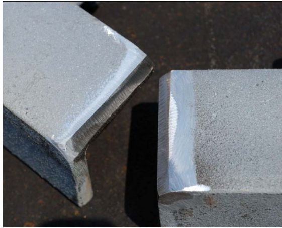
Both pieces beveled and coating next to weld zone removed.
