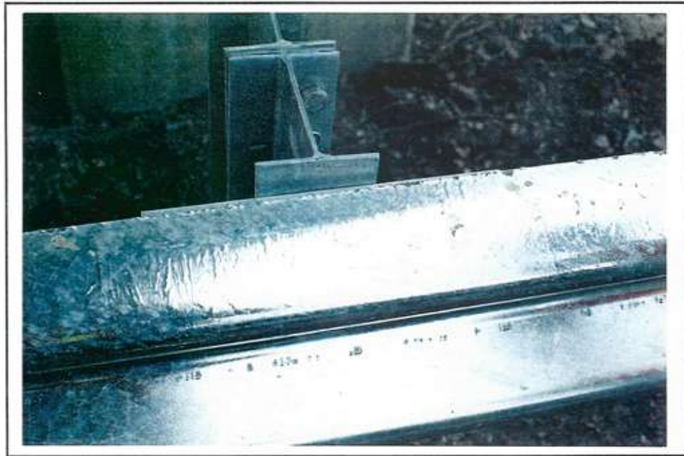
Photo 39 Condition: Bare Spots (Exposed Steel)
