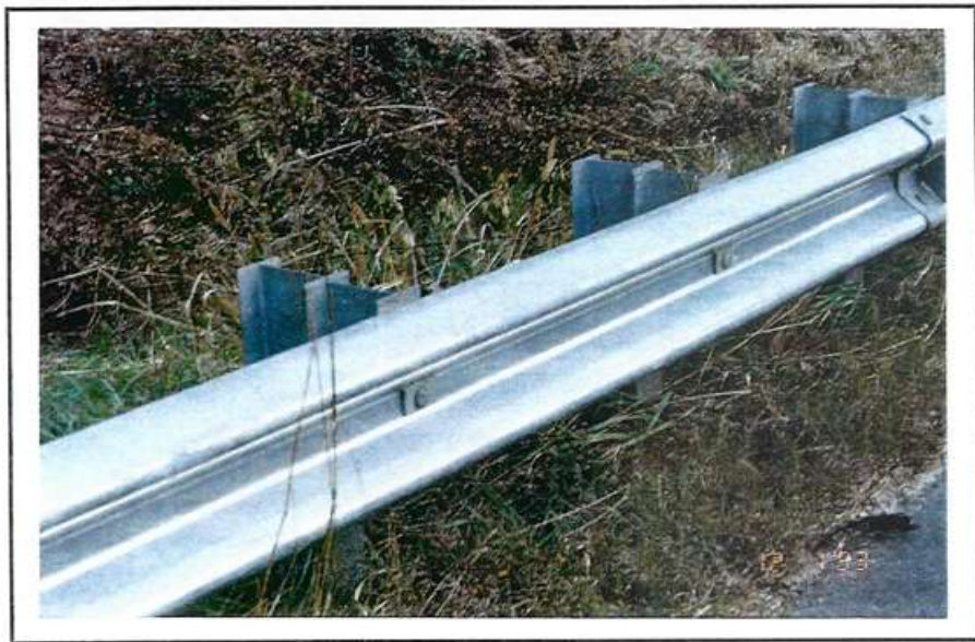
Photo 93 Example of good guardrail.
