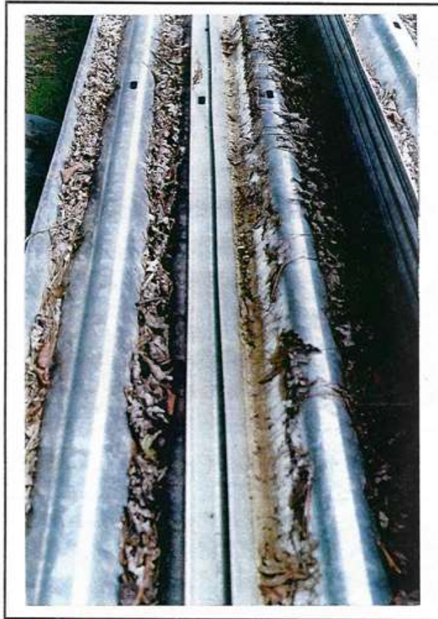
Photo 83 Improper storage. The leaves will help keep moisture on the items and they will also decay adding to the corrosion process.
