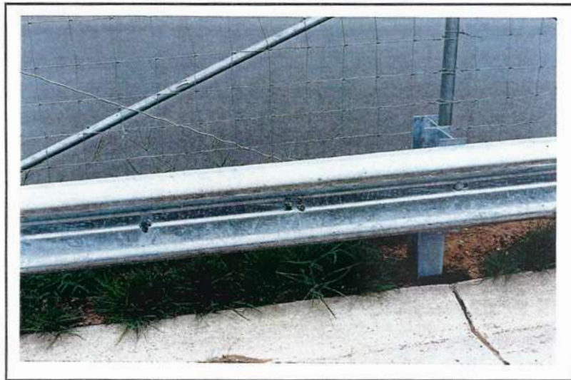
Photo 66 Condition: Flux Inclusion
