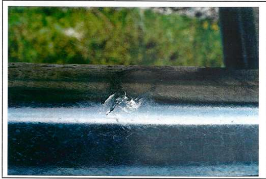
Photo 51 Condition: Ash Inclusions
