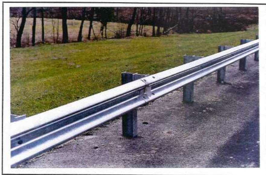
Photo 95 Example of good guardrail.
