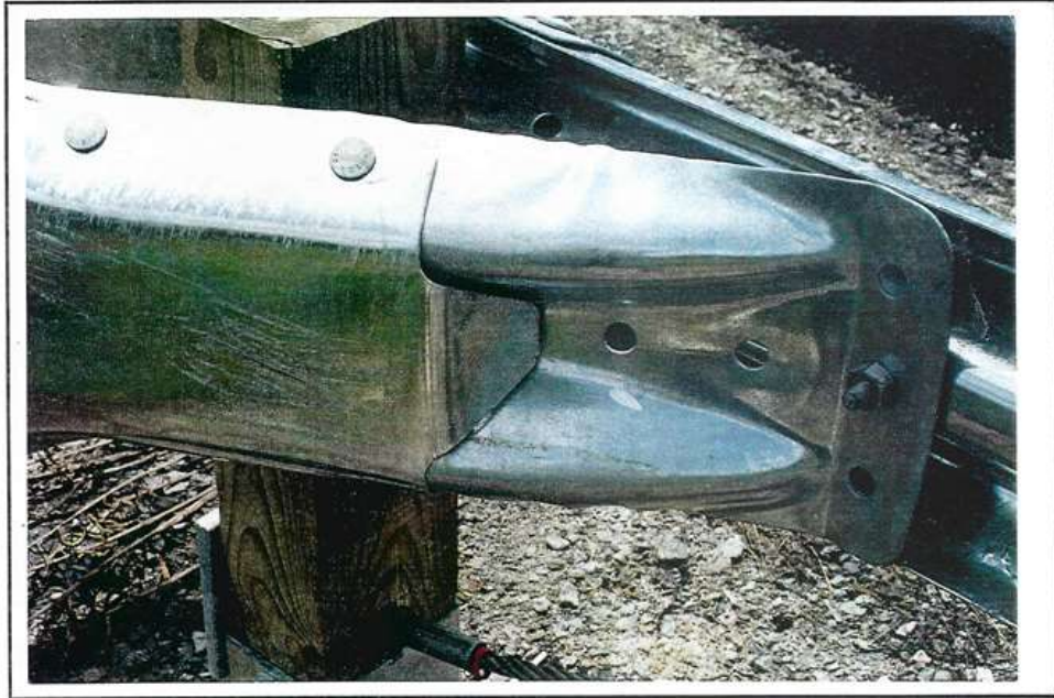
Photo 92 Example of good guardrail.
