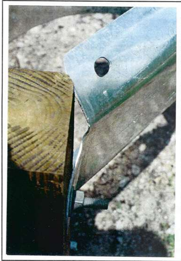
Photo 64 Condition: Field Bending (Field Fabrication)
