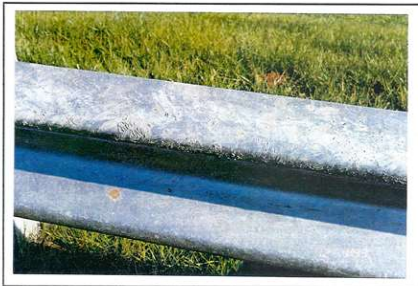
Photo 52 Conditions: Excessive Ash Inclusions
