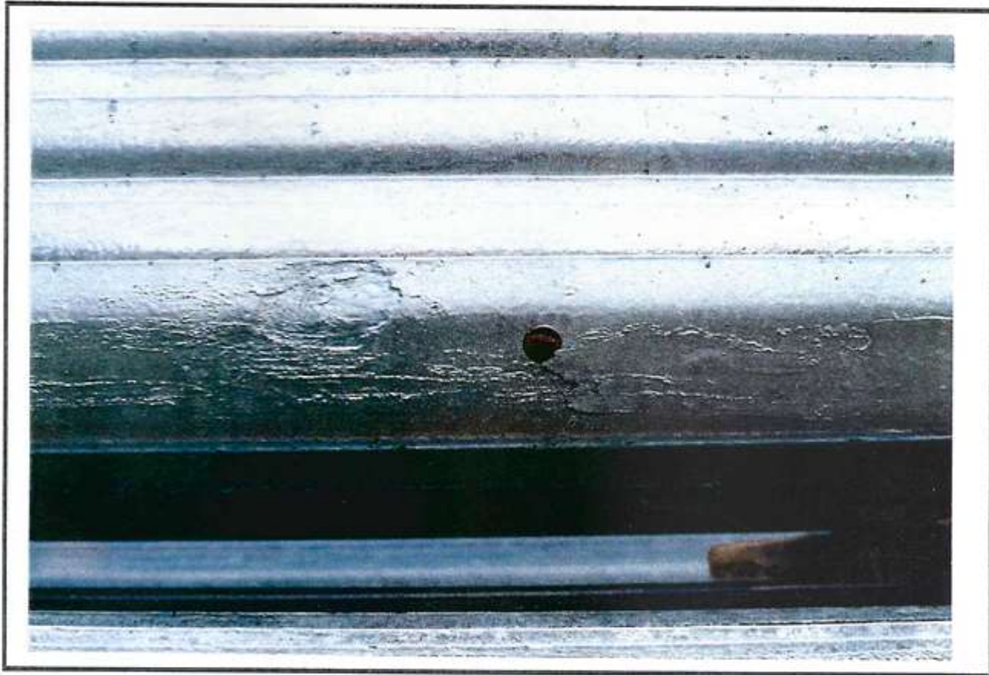
Photo 71 Condition: Laminations
