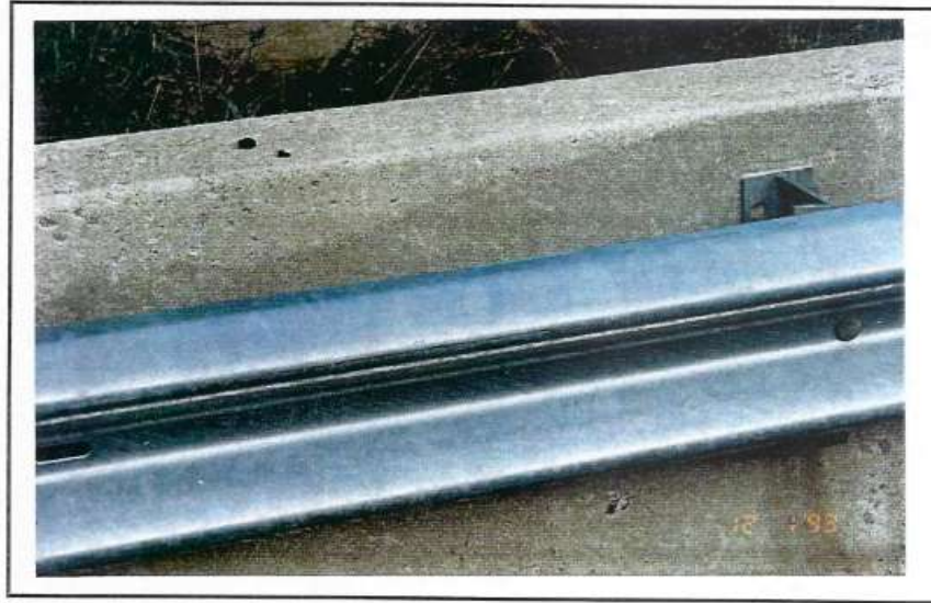
Photo 94 Example of good guardrail.
