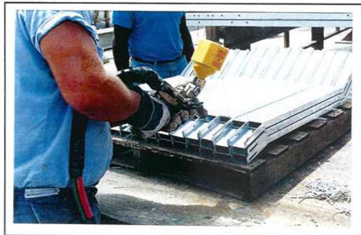
Photo 44 Bare spots on galvanized material being repaired at the producer's yard.
