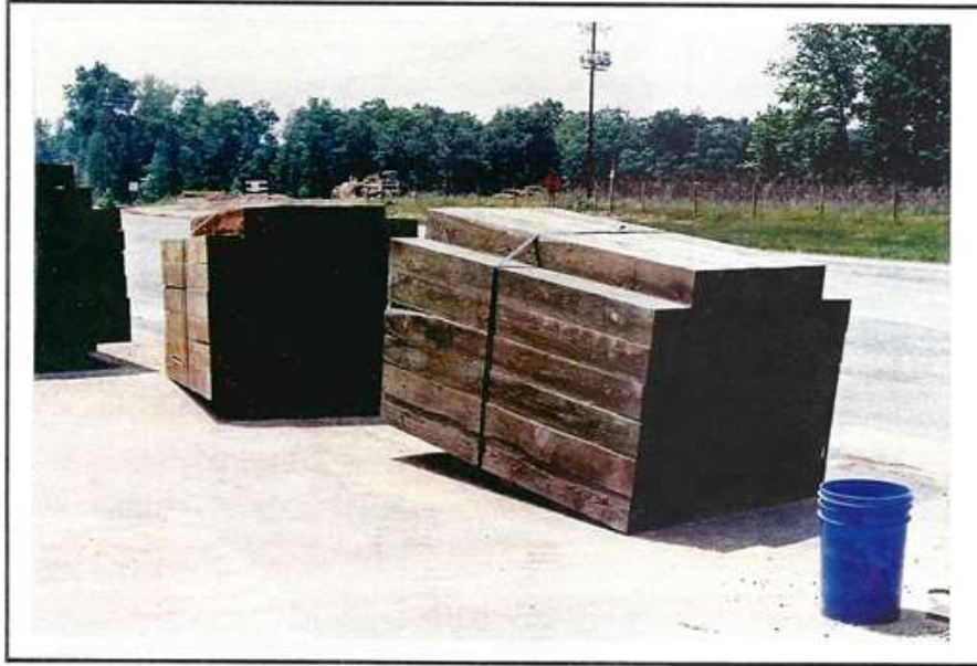
Photo 78 Wood guardrail posts. Notice the blue bucket of nuts and bolts. They should be stored in closed containers to keep moisture out.
