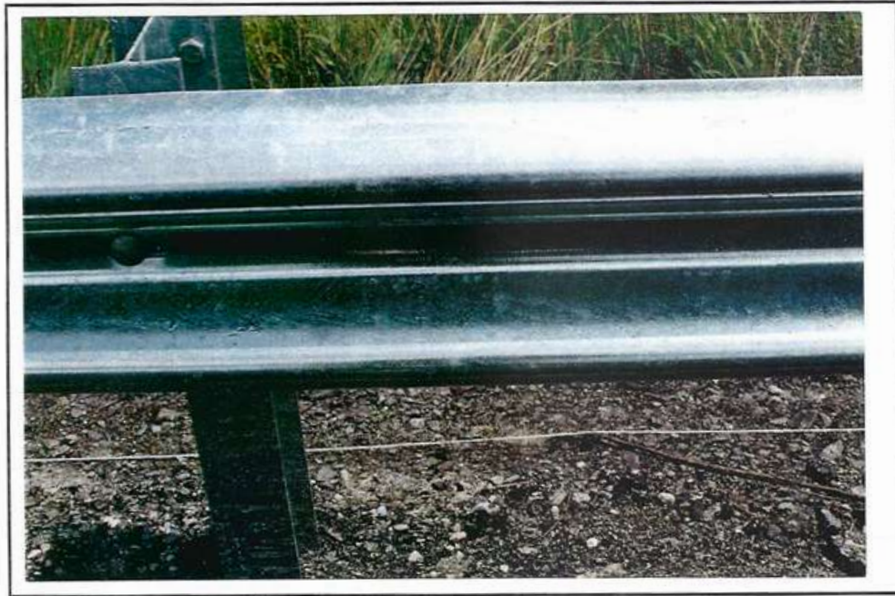
Photo 91 Example of good guardrail.
