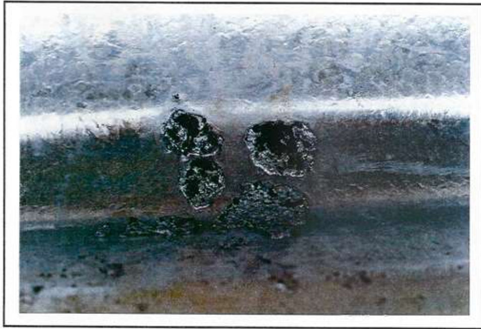
Photo 47 Condition: Ash Inclusions
