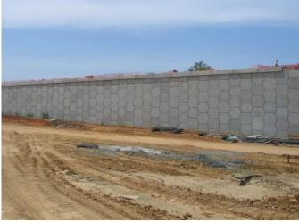
Figure 1: Example of a MSE Wall
