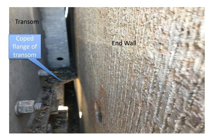
Verify clearance from the end wall to the transom beam. Typically the transom beam is coped.
