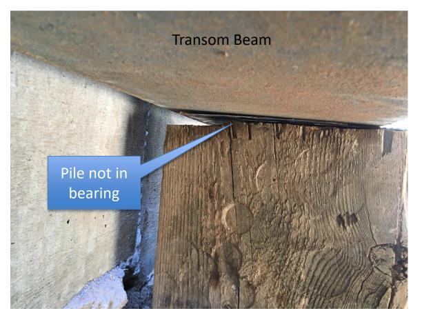
Bolster detail showing timber on H-Pile
