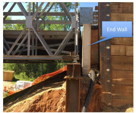
Verify clearance from the end wall to the transom beam. Typically the transom beam is coped.
