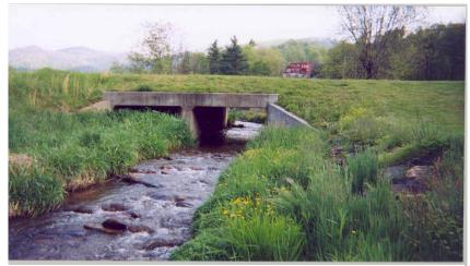
Figure 3. Culvert with Floodplain Bench
