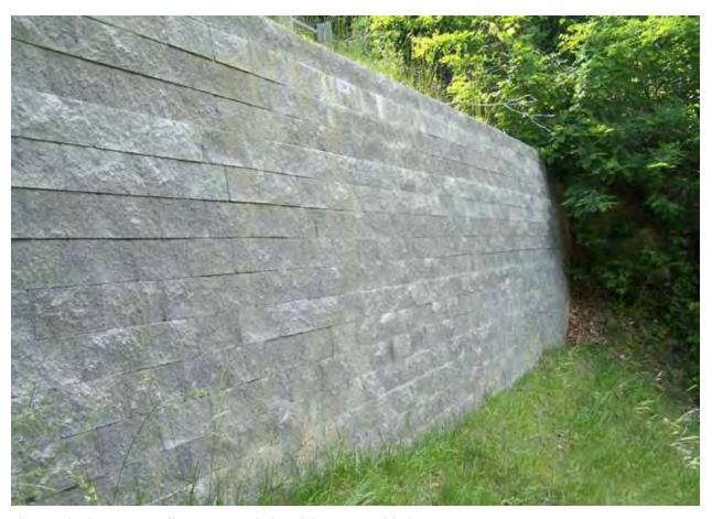
This standard retaining wall is constructed of modular concrete blocks. Image courtesy NCDOT.
