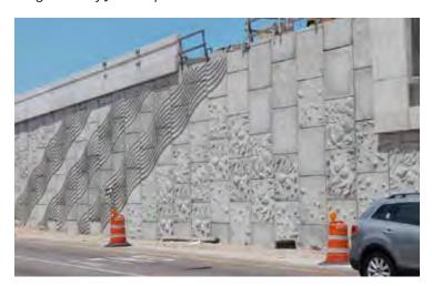
Wavy diagonal lines and patterns that look like shells and other sea elements are used for a precast concrete retaining wall at the intersection of US 19 and SR 60 in Clearwater, Florida. Image courtesy Creative Design Resolutions.
