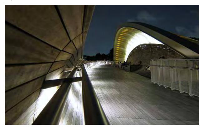
The curved ribs of Henderson Waves Bridge form alcoves that provide seating when needed for public events. Image courtesy of Wikipedia Commons.
