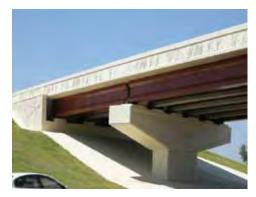
The bridge for US-77 over I-35 in Norman, Oklahoma, includes decorative details such as emblems on the abutments and horizontal rails, a styled pier, and red girders to add visual interest. Image courtesy Creative Design Resolutions.
