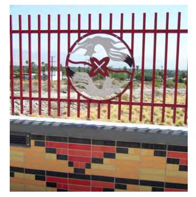
Enhancements to the Bob Hope Interchange on I-10 have made Basket Bridge into a landmark for the Agua Caliente Band of Cahuilla Indians' nearby casino. Braaksma Design Inc researched the Tribe's heritage and desert environment to present images for incorporation into the bridge railing, piers and sloped paving. The basket patterns and plant motifs that are fabricated from galvanized mesh and powder-coated steel, celebrate the Tribe's basket-making tradition.
