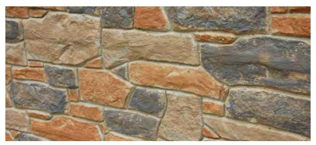
The stone treatments for the new bridge at Exist 104 - Enola Road that crosses Interstate 40 are created using form liners. The patterns created from the form liners were then stained to create a more natural -looking stone pattern. The columns use an attractive modular pattern that creates strong, simple lines. Image courtesy NCDOT.
