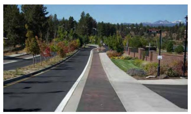
Along US Highway 97 in Bend, Oregon, are stained walk/bike trails, raised medians with native plant materials, a meandering road geometry to maintain a pedestrian scale, and lighting for security and safety. Image courtesy Oregon DOT.
