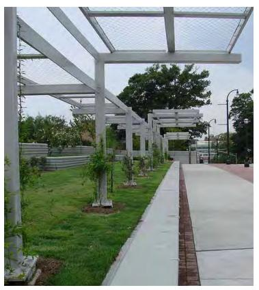
This overhead structure provides visual interest for this overpass. The overhead trellis will eventually be covered by the vines planted at the base of each post. This will soften the impact of the structure and create a more inviting pedestrian walk. Image courtesy EDAW.
