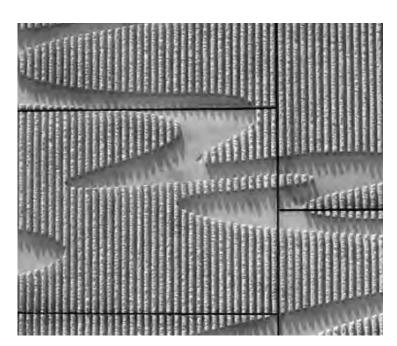
This is an example of precast concrete panels that fit together to create a wave pattern. The combination of the wave pattern and the variations in texture with the groved vertical lines in the foreground and the smooth texture in the background help create visual interest. Image courtesy FHWA.
