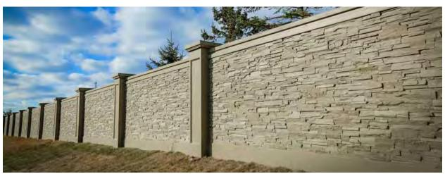
This precast concrete noise wall uses a fieldstone pattern on the panels, a shadow box and cap on columns, and a smooth pattern for the base and cap of the panels to add visual consistency and continuity. All of the components are a light grey, which helps reduce the visual dominance of the wall. Image courtesy James Sipes.
