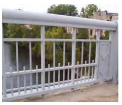
The small size of the bars makes it easier to see the river from the bridge. Image courtesy FHWA.
