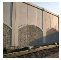
Construction for this concrete retaining wall is nearing completion. Form liners were used to create the patterns. Image courtesy FHWA.
