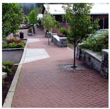
This pedestrian walkway in Lake Oswego, Oregon, is a good example of an enhanced walk. The use of brick pavers, concrete curbs and accessibility ramps, tree grants, retaining walls, and variety of landscaping all help create a comfortable, inviting pedestrian space. Image courtesy PBIC Image Library and Dan Burden.
