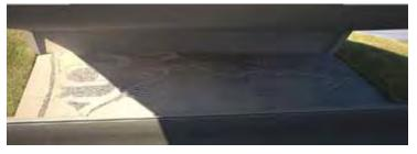
The paved areas underneath the Stockton Delta Bridge in Stockton, California, have added detail created by concrete form liners. Image courtesy Creative Design Resolutions.
