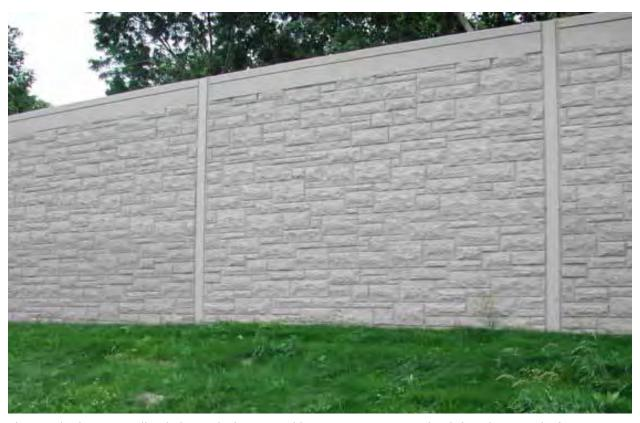
This standard NCDOT wall includes steel pilings, an ashlar stone pattern created with form liners, and a faux top created by a smooth surface along the top of the wall. Image courtesy James Sipes.
