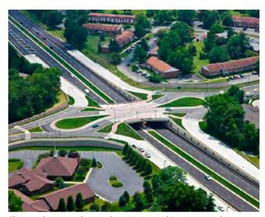
This teardrop interchange along US 64 combines improved functionality while also enhancing aesthetics by the use of strong curvilinear lines and the combination of patterns and textures. Image courtesy FHWA.
