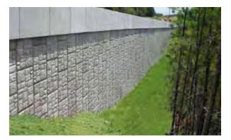
Precast concrete panels with a stone pattern on the surface was used to create this retaining wall for the McGinnis Ferry Road Extension in McGinnis, Georgia. Existing vegetation was preserved in order to reduce the visual impact of the wall on adjacent land uses. Image courtesy James Sipes.
