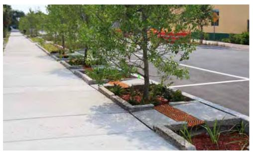
The sidewalk on Deadrick Street in Nashville, Tennessee, is separated from the street by a series of planters that are linked together to create an urban bioswale. Image courtesy EDAW.
