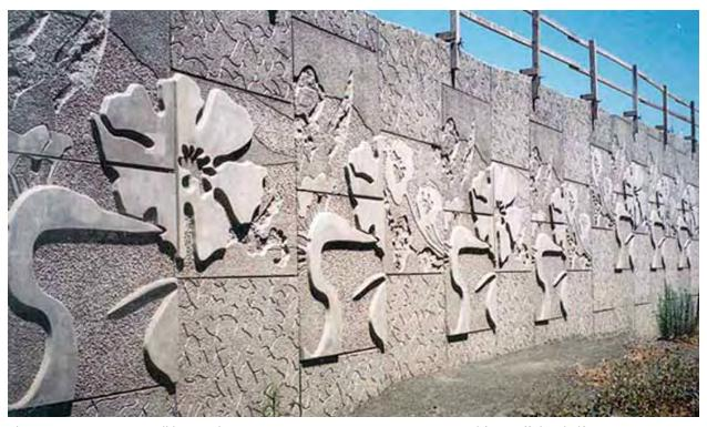
This concrete retaining wall by Braaksma Design Inc uses custom images created from off-the-shelf textures.
