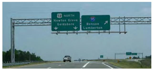
A standard sign gantry on I-295 is used to support directional signage for 13 North and I-95. The small size of the metal components, openness of the horizontal elements, and light gray color of the structure helps reduce the visual impact of the gantry. Image courtesy NCDOT.
