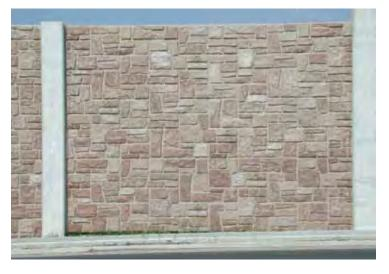
A rustic ashlar stone pattern stained to create a darker surface is outlined by smooth concrete piers. There is no cap along the top of the wall. Image courtesy Customrock.
