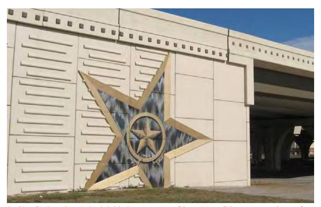
For this wall in Texas, Texas DOT included the Texas Star as part of the retaining wall that serves as an abutment for this bridge. The wall is made of MSE modules that ether have a smooth surface or offsetting horizontal bars to add visual interest. The Star is part of seven different MSE modules. Image courtesy Customrock.
