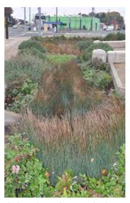
This bioswale uses plant material, soil improvements that encourage infiltration, weirs, and grading to control stormwater runoff. Rougher textures help slow down runoff. Image courtesy Mike Houck.
