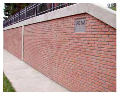
A used brick form liner is used for the surface of this wall. Image courtesy EDAW.
