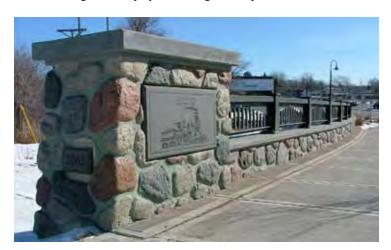
This wall with the railroad sign includes a Minnesota fieldstone form liner pattern and metal rails. Image courtesy Customrock.
