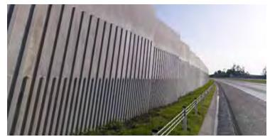
This noise wall in Bonville, New South Wales, is at a slight angle so that adjacent panels have an offset from the previous panel. An angular pattern is used to decorate the wall. Image courtesy EDAW.
