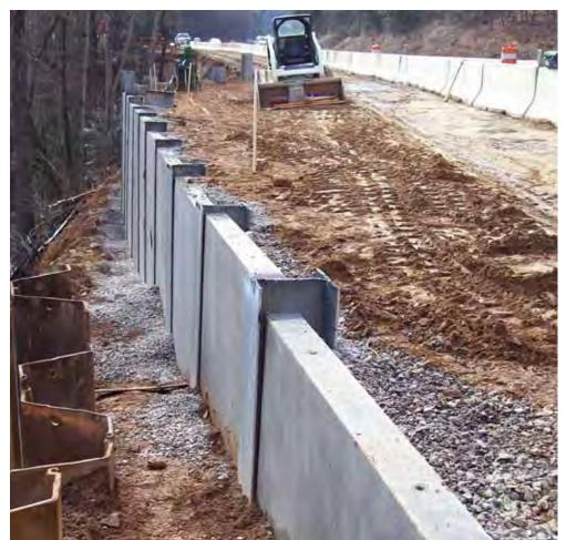
These retaining walls constructed of steel piers and precast concrete panels are used to stabilize slopes along North Carolina roadways. Emphasis is more on functionality than aesthetic appeal. Image courtesy NCDOT.
