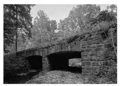
The Otter Creek Bridge on the Blue Ridge Parkway is constructed of stone faced arches that mimic rigid frame structures. Image courtesy FHWA.
