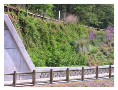
This is another example of using native materials to create a green wall along the grade separation of the roadway and a multipurpose trail. Image courtesy EDAW.
