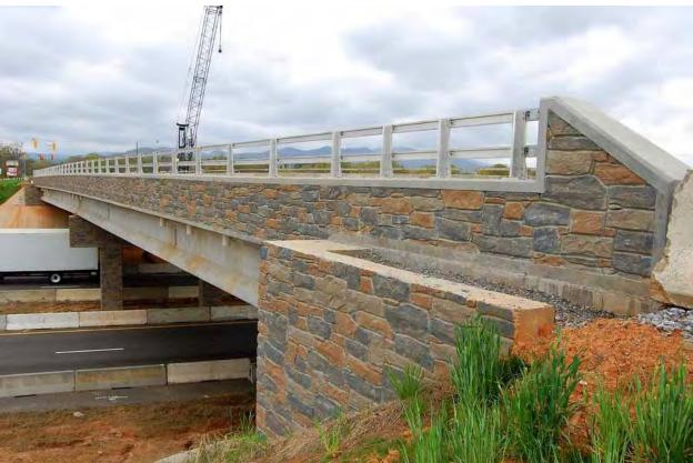
NCDOT replaced the bridge at Exist 104 for Enola Road that crosses Interstate 40. The City of Morganton , North Carolina, worked with NCDOT to design and fund enhancements to this bridge, including stone treatments to the retaining walls, bridge rails, and columns visible from I-40. Images courtesy NCDOT.
