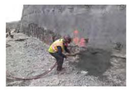
Contractors are using shotcrete to complete the structural construction phase of a wall below the Food Lion on US 321 in Blowing Rock North Carolina. Image courtesy NCDOT.
