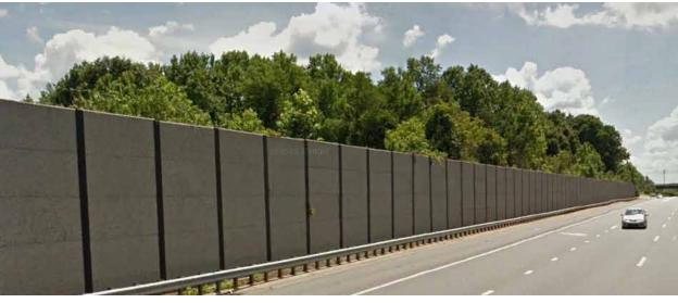
These are examples of Standard Noise Walls used along North Carolina roadways. Both use a pier and panel approach for wall construction. Images courtesy NCDOT.
