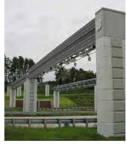
The toll gantries for the Triangle Expressway allows cars using an NC Quick Pass to use the road without slowing down to pick up a ticket or pay a toll. All cars are required to have an NC Quick Pass. Image courtesy James Sipes.
