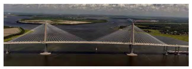
The Arthur Ravenel Jr. Bridge, near Charleston, South Carolina, uses a cable-stayed suspension design with two diamond-shaped towers. Each tower is 575 feet tall, and the combination of towers and cables help make this a landmark bridge. Image courtesy David Oppenheimer.
