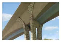
This is a close-up view of the stone-formed central columns for the Bridge to Nature that are intended to reflect the natural stone found in Vermont. Image courtesy Vermont Transportation.
