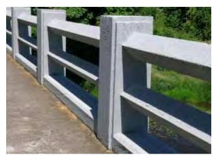
Massive geometric concrete rails are used on the Brownsville Bridge, Texas. Image courtesy FHWA.
