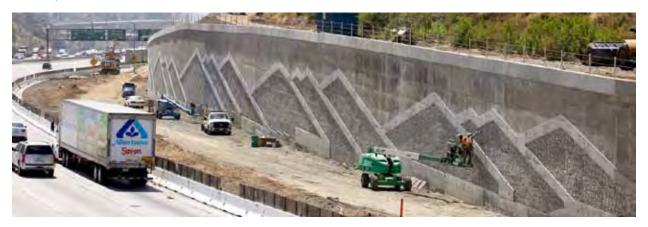
This large retaining wall uses a mosaic of mountain peaks created with form lined concrete to add visual interest and break up the perceived scale of the wall. Image courtesy FHWA.
