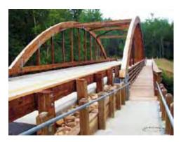
A wooden arch bridge in North Carolina also has wooden guard rails and posts for the pedestrian walkway so there is a visual consistency for all the design elements. Image courtesy FHWA.
