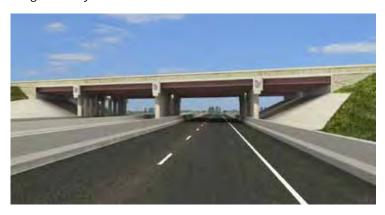
The Garth Brooks Bridge in Canadian County, Oklahoma, is design with strong horizontal lines, details on the columns on horizontal members, and darker girders to help add a sense of depth. Image courtesy Creative Design Resolutions.
