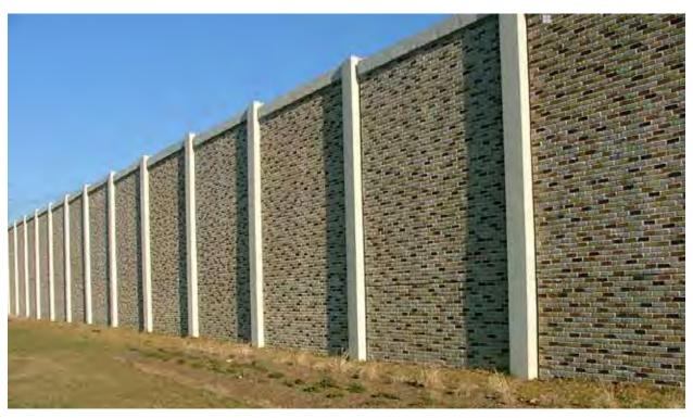
This wall is constructed of light-colored concrete piers and cap, and precast panels created with used brick form liner. Image courtesy Customrock.
