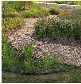
Gravel was used to emulate the meandering flow of a stream as part of this bioswale. Image courtesy AECOM.
