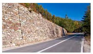
Despite its height, this retaining wall is not visually objectionable because the stone veneer reduces the perceived scale of the wall. Image courtesy DepositPhotos.com.
