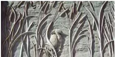
This image of a crane and wetland vegetation was created on a panel using form liners. This panel can be used as part of noise walls, retaining walls, or other structural elements. Image courtesy Liz Pope, Scott Systems.
