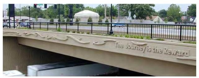
The Kellogg Oliver Bridge in Wichita, Kansas includes decorative elements along the bridge span and metal rails along the top of the bridge. Image courtesy Creative Design Resolutions.
