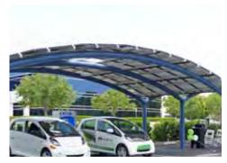
This overhead shelter includes solar panels that help charge these electric cars. Image courtesy EDAW.
