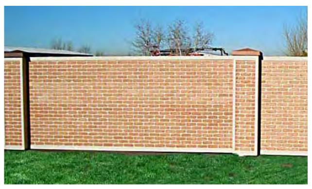
This is a standard concrete noise wall with form liners used to create the appearance of bricks. The lighter colors on the columns and along the top and bottom of the walls visually fits the 'grout' lines in the panels. Image courtesy FHWA.
