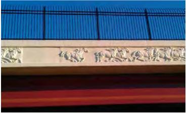
Rock Creek Road which crosses I 35 in Norman, Oklahoma, includes reddish girders, detailed frescos on the horizontal parts of the bridge, and metal railings along the top to serve as a barrier for pedestrians. Image courtesy Creative Design Resolutions.
