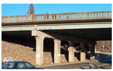
This bridge abutment has a stone pattern surface to add visual interest by using a finer texture and warmer color. Image courtesy NCDOT.
