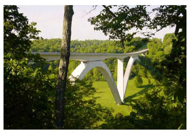
The Natchez Trace Parkway Bridges is a double-arch bridge that spans across Highway 96 near Nashville, Tennessee. It's located at mile marker 438 on the Natchez Trace Parkway. The bridge was completed in 1994, and is the first segmentally constructed concrete arch bridge in the United States. Image courtesy FHWA.
