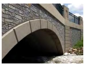
This wall uses a minnehaha blend form liner to create the appearance of stone. Image courtesy Customrock.
