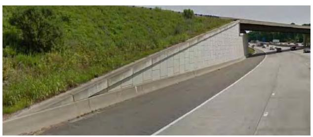
These retaining walls are used to create bridge abutments that structurally support the bridge over the roadway and stabilize the adjacent slopes. These walls are made of modular MSE panels outlined by concrete caps. A standard jersey barrier is located in front of the wall. Image courtesy James Sipes.
