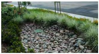
Gravel is used to slow down stormwater runoff in this bioswale, and the plants filter sediment and pollution runoff. Image courtesy EDAW.
