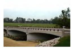
On Paris Pike, which connects Paris, Kentucky, to Lexington, Kentucky, the new bridge over North Elkhorn Creek has a low profile that blends with the landscape. The light gray concrete, stone abutments, simple columns, and open rail are all part of the bridge aesthetics. Image courtesy Wikipedia Commons.
