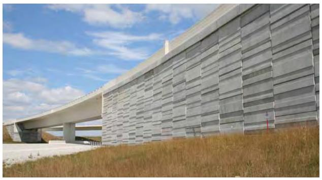
The retaining walls that make up the abutments for this bridge along I-70 near the Indianapolis Airport are constructed of reinforced earth MSE precast retaining wall. The smooth texture and while color of the bridge and railings visually fit with the light to medium gray panels that look a bit like slate. Image courtesy INDOT.
