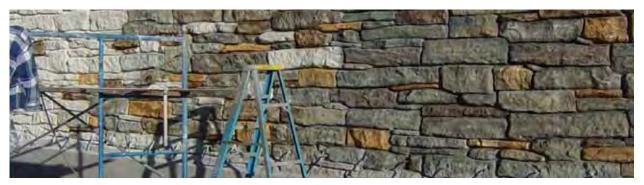
This image shows how a wall created with a form liner is being stained by hand to create a more realistic appearance of the stone. Image courtesy NCDOT.
