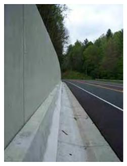
These images show Standard bridge abutments (very top & right) that are poured-in-place concrete that stabilizes the slopes, with plantings along the sides, The image above shows a Standard concrete retaining wall along a roadway. Image courtesy larges Sings courtesy James Sipes.
