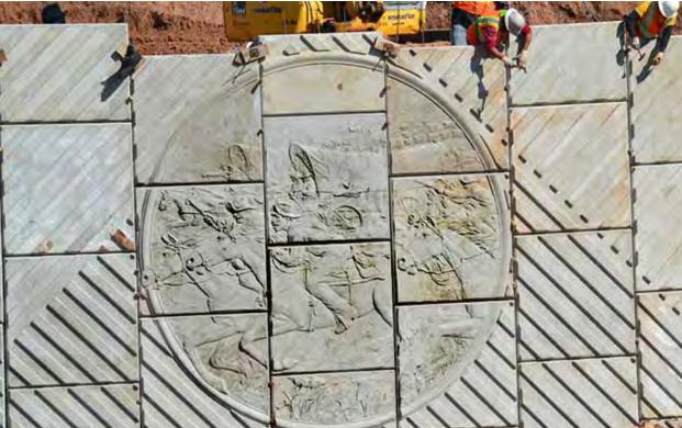
This abutment on the Main Street Bridge in Norman, Oklahoma, includes diagonal patterns, a stone cap, and large round images showing the Oklahoma Land Rush that occurred in 1889. Image courtesy Creative Design Resolutions
