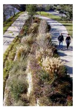
This bioretention area helps reduce sedimentation and stormwater runoff into this river in Austin, Texas. Image courtesy PBIC Image Library and Dan Burden.
