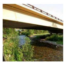
The Jocko River Bridge along U.S. 93 on the Flathead Indian Reservation in northwest Montana is simple in design so it doesn't distract from the surrounding landscape. It is also designed with sufficient height and span to allow for the continuation of ecosystems and the crossing of wildlife. The incorporation of wildlife considerations makes this bridge a more integrated solution than is normally used. Image courtesy MTDOT.
