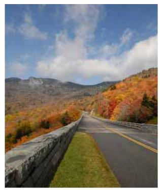
This view of Blue Ridge Parkway shows the use of stone retaining walls, narrow shoulders, and a limited right of way to minimize impacts on the surrounding landscape. Image courtesy FHWA.
