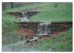
These stone weirs are used to slow down stormwater runoff and prevent scouring. The stone walls also create a more attractive setting. Image courtesy EDAW.
