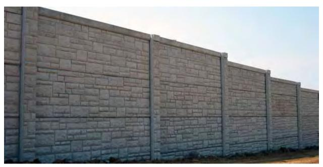
This ashlar stone finish noise wall includes a reflective facing. This side of the wall is on the residential side of the development. Image courtesy NCDOT.
