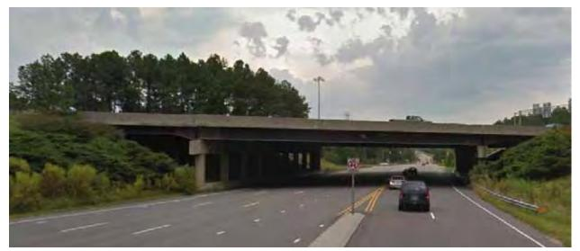
The Page Road bridge is a steel plate girder bridge and is one of several types of standard NCDOT bridges. Image courtesy James Sipes.
