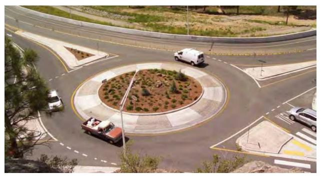
This diamond roundabout helps direct traffic while keeping automobiles moving. The planting, sculpture, and changes in paving pattern in and around the roundabout is intended to soften the visual impact of the paving. Image courtesy Colorado DOT.
