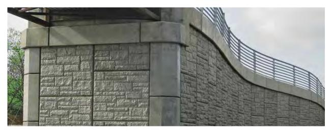
This bridge abutment is constructed of MSE panels with form lined stone pattern surfaces. Image courtesy James Sipes.
