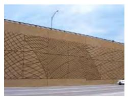
Retaining walls along US 54 through Wichita, Kansas, use a darker earthtone stain and wavy patterns to provide visual interest while also reducing the visual impact of the wall. Image courtesy Creative Design Resolutions.
