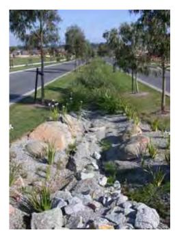
This bioswale is located within a roadway median in Lynbrook, Australia. The combination of plant material, gravel, and larger rocks helps management stormwater runoff in a manner similar to natural systems. Image courtesy AECOM.
