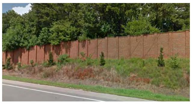
This brick noise wall is installed along U.S. 540 in Raleigh, North Carolina. The mature vegetation behind the wall and the newer vegetation in front help reduce the visual impact of the wall. Image courtesy James Sipes.
