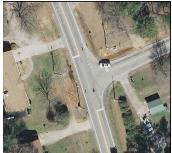
Top: Signalized intersection with left turn lanes; Bottom: Signalized intersection without left turn lanes
